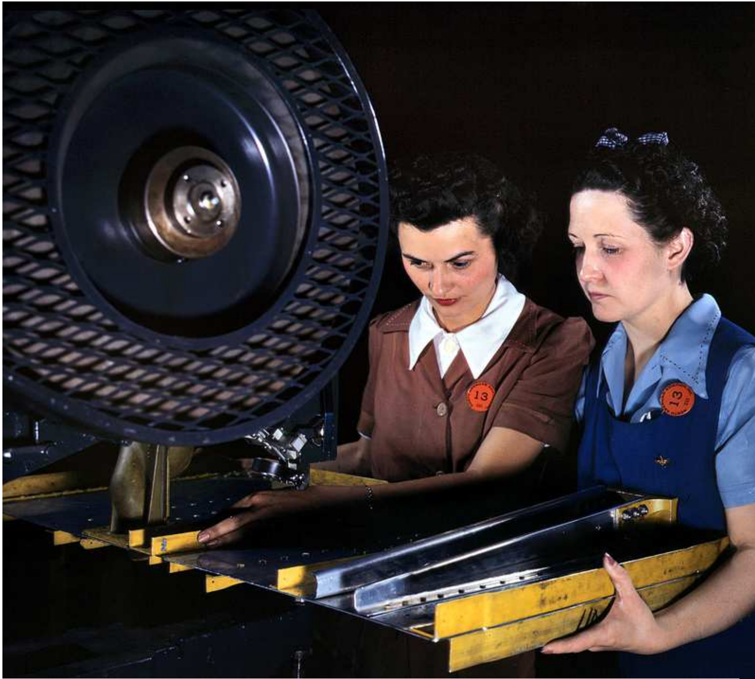
June 1942. Inglewood , California . "Punching rivet holes in a frame member for a B-25 bomber at North American Aviation." 4x5 Kodachrome transparency by Alfred Palmer for the Office of War Information.
